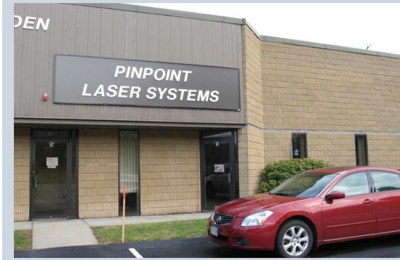
Pinpoint Laser Systems Facility
